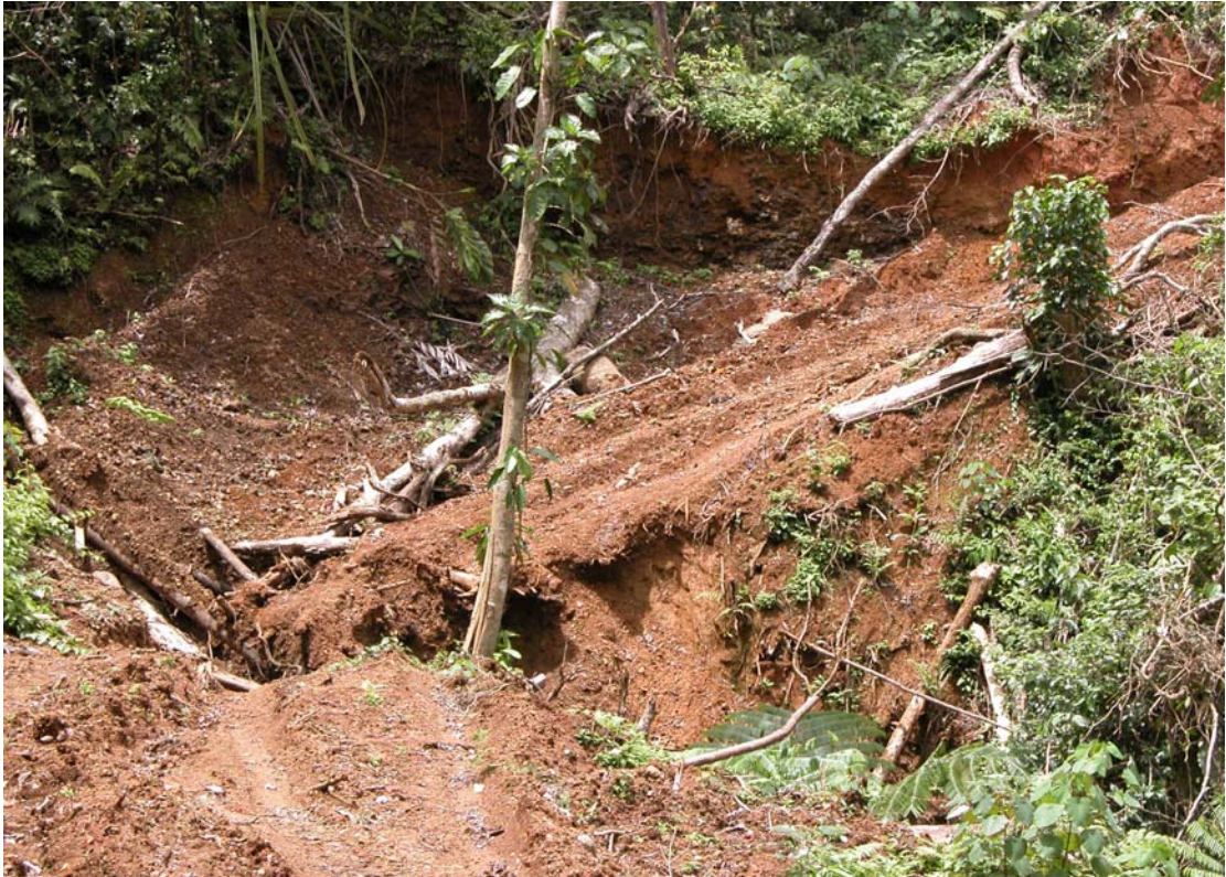
Logging roads cause accelerated soil erosion, especially when designed poorly (WCS).
